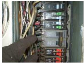
contractor at this time to prevent any possibility of future malfunctions. The conductors that are double tapped are under sized in ratio to over current protector which could cause electrical wires to overheat and pose a fire hazard.
