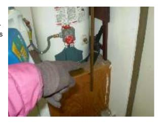
BRACING: The water heater tank is not properly braced per California requirements
