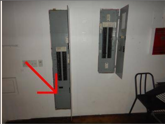
Suspected overheating of incoming feeder.
