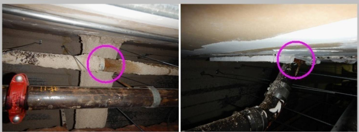
8th floor hall above ceiling tiles
