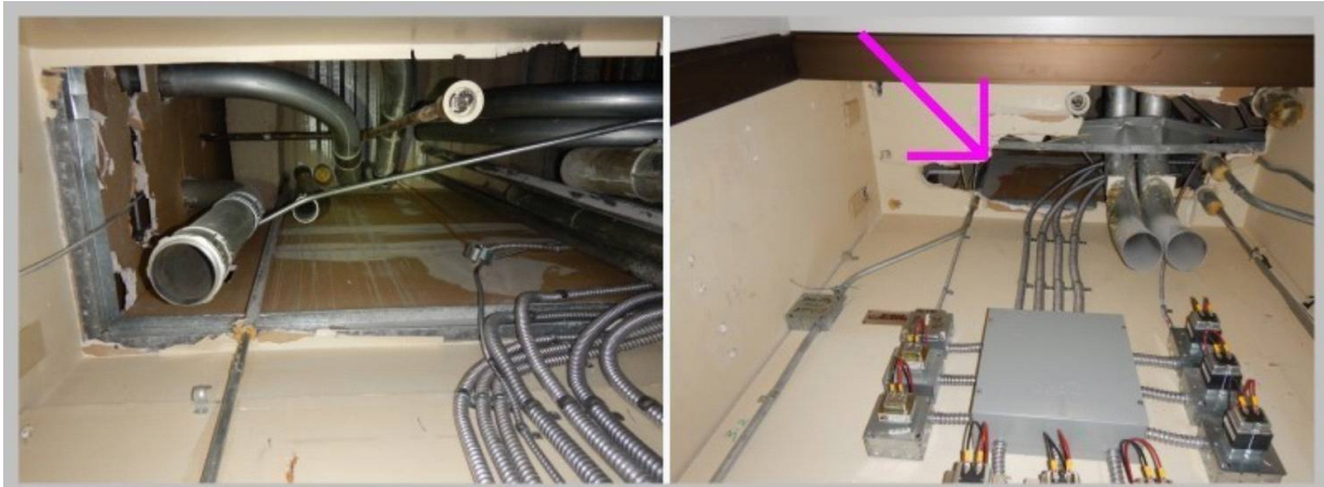
2nd & 3rd Floor Men's restrooms
