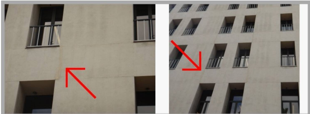
Stucco cracks
